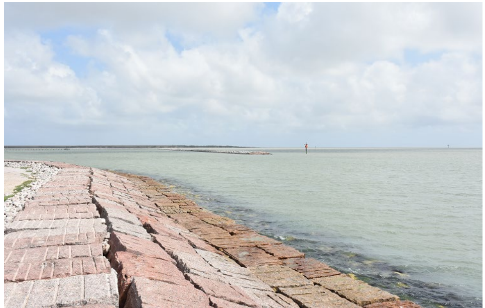
Figure 13: Photograph of revetment.
